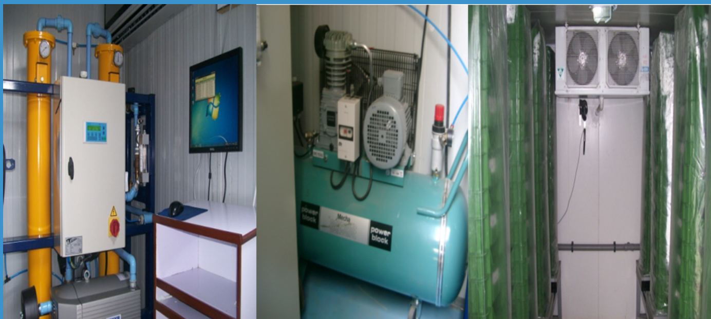
CA system (L-R): Nitrogen generator, Compressor, Cold store with temperature and relative humidity control
